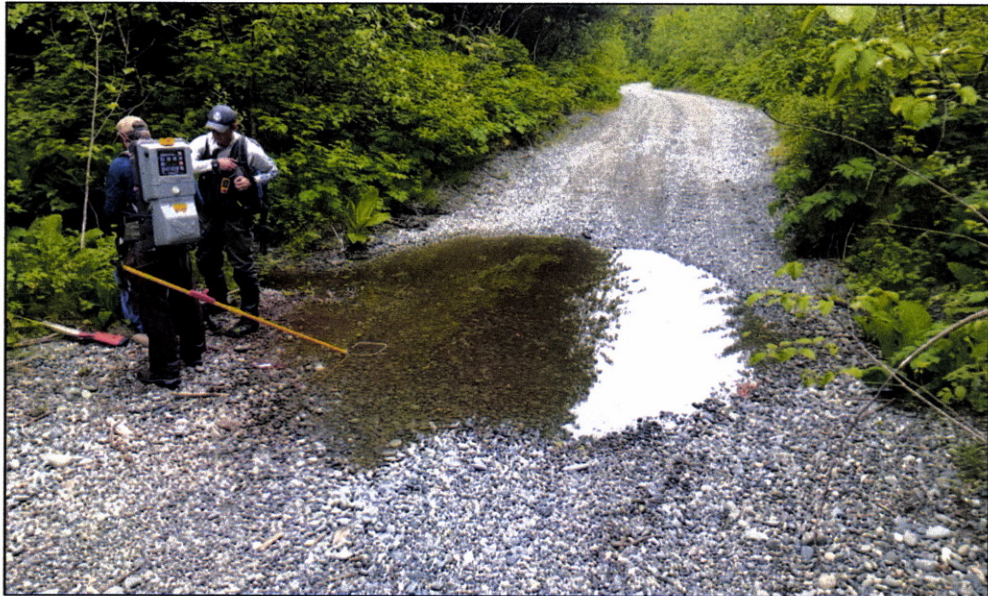
Figure 4.—Impounded water on the road at waypoint 265.
