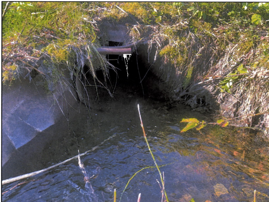
Figure 3. —Culvert upstream of the road.
