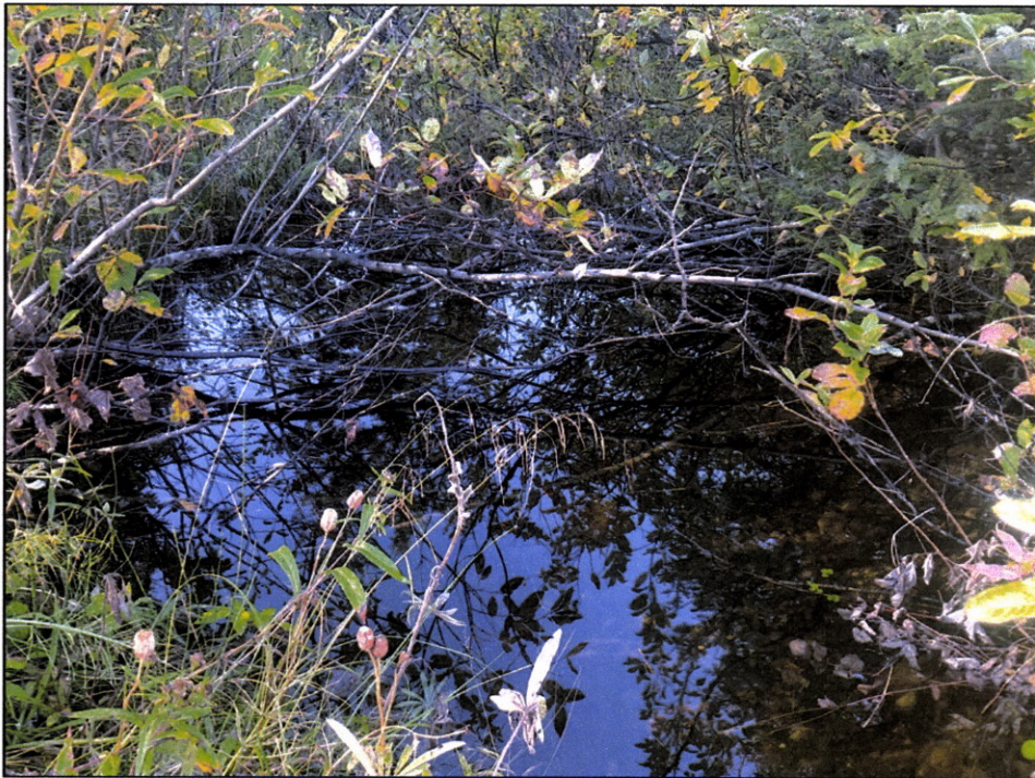
Figure 3. —Ponded water upstream of the culvert.
