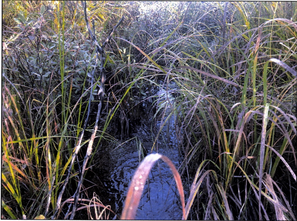
Figure 2.—Channel downstream of the culvert.
