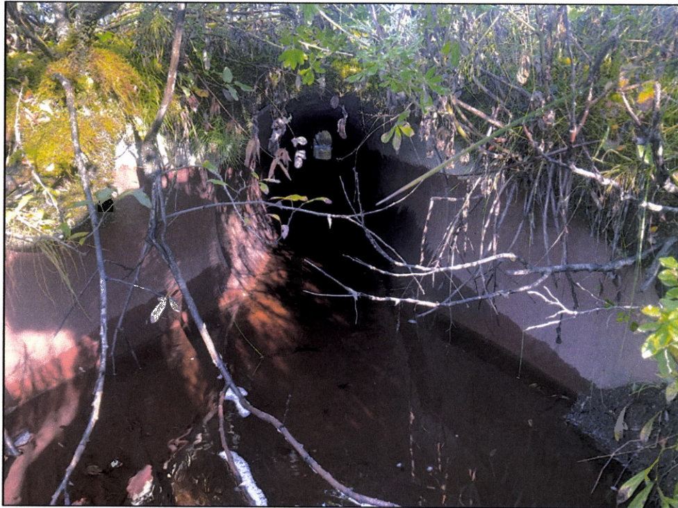
Figure 3.—Culvert downstream of the road.
