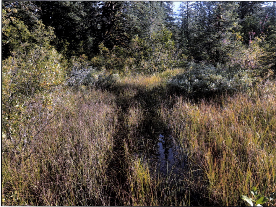
Figure 2.—Channel downstream of the culvert.
