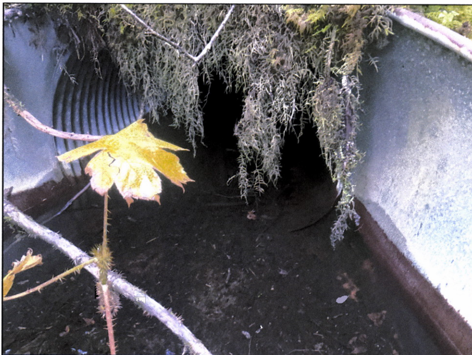
Figure 3.—Culvert downstream of the road.
