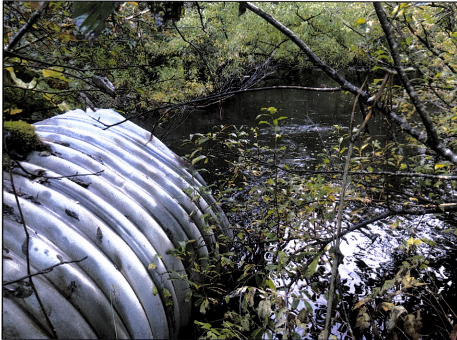
Figure 2.—Channel downstream of the culvert.
