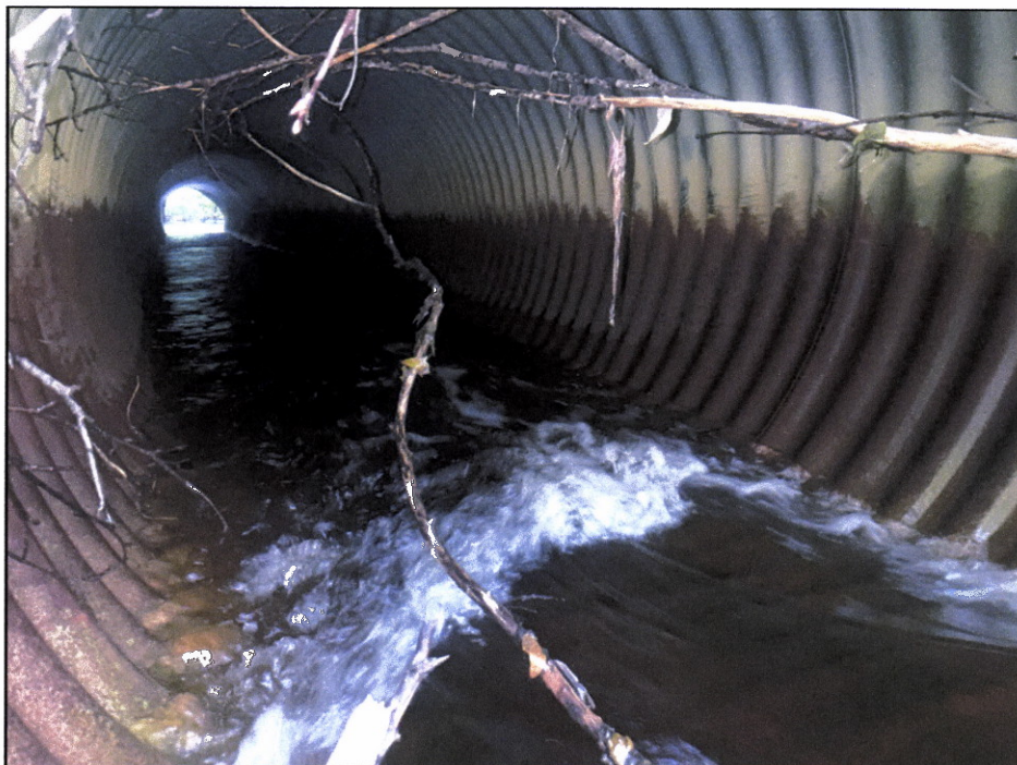
Figure 3.—Inside of culvert looking downstream.
