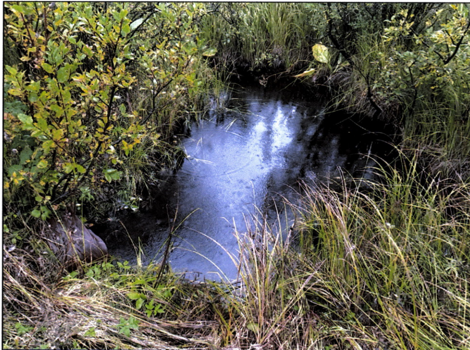
Figure 3.—Culvert upstream of the road.
