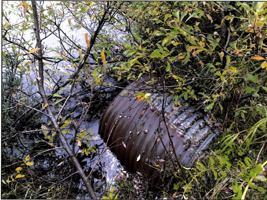
Figure 2.—Inlet of culvert at waypoint 1237.
