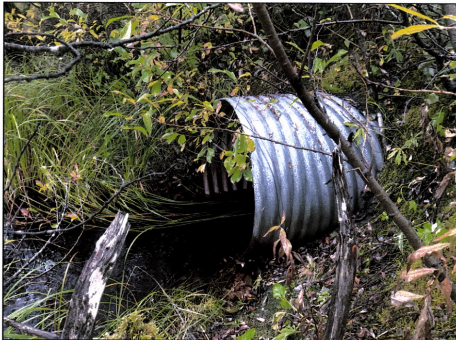
Figure 3.—Culvert upstream of the road at waypoint 1242.
