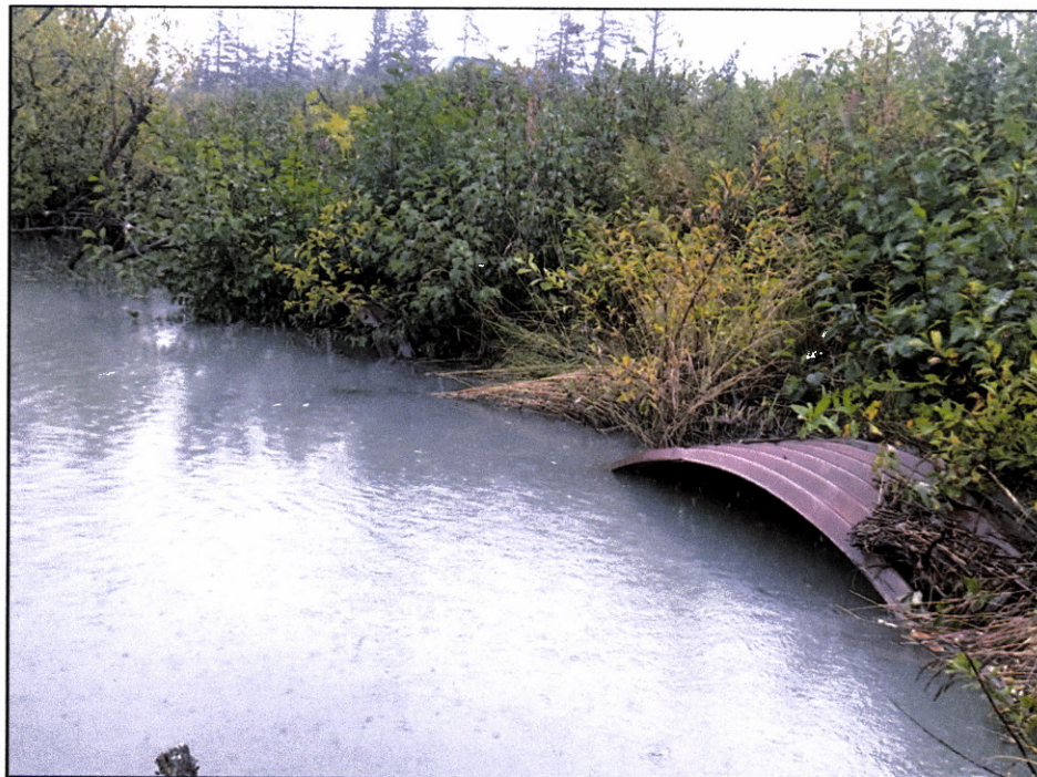
Figure 3.—Twin culvert inlets.
