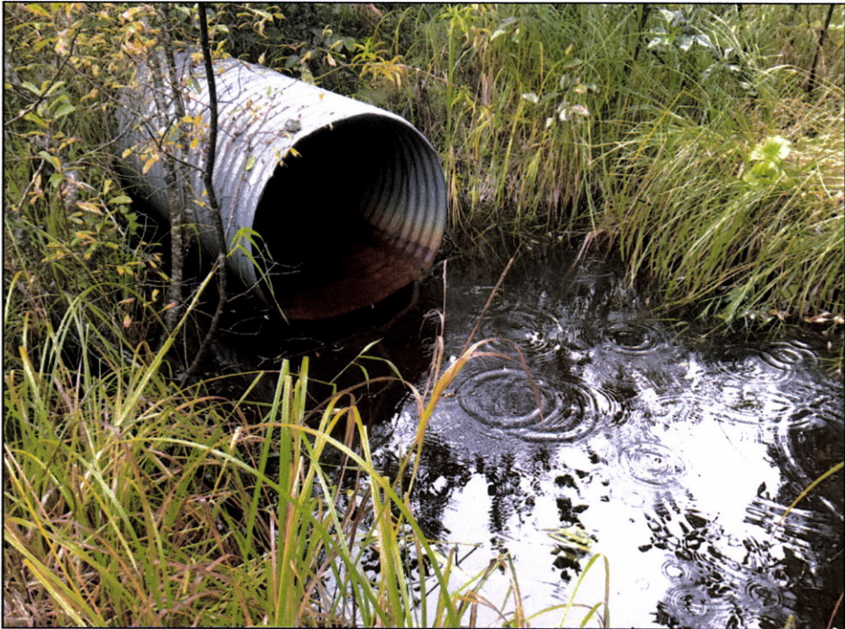
Figure 3.—Culvert at waypoint 1245
