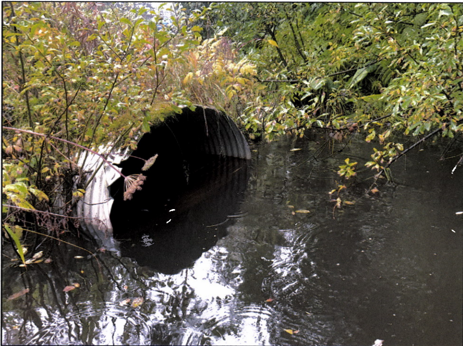
Figure 3.—5ft culvert at waypoint 1248.
