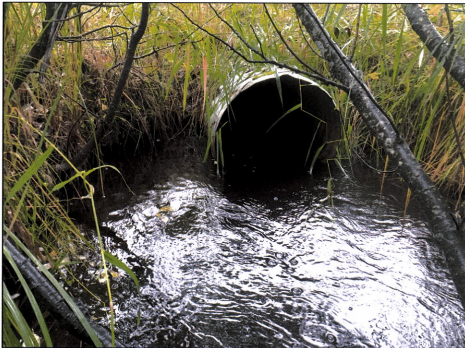
Figure 3.—Culvert at waypoint 1246.
