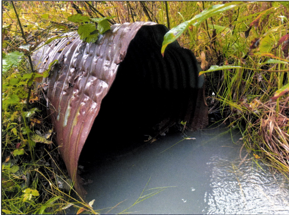
Figure 2.—Culvert inlet at waypoint 1249.
