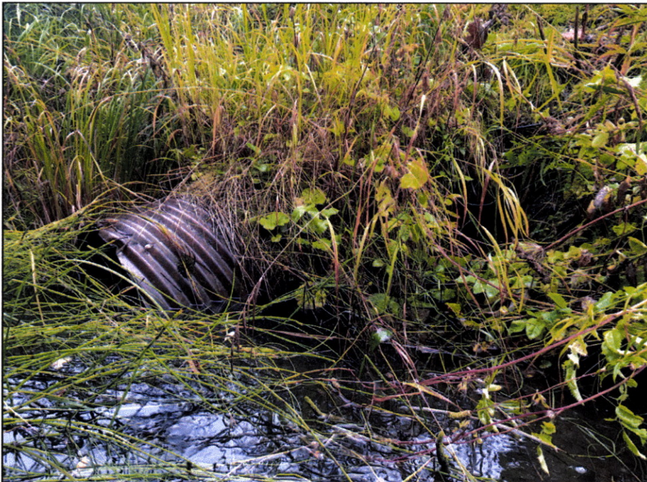
Figure 3.—Culvert outlet at waypoint 1249.
