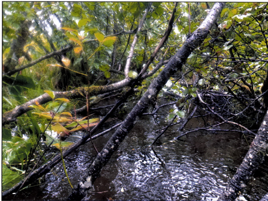
Figure 3.—Culvert at waypoint 1245
