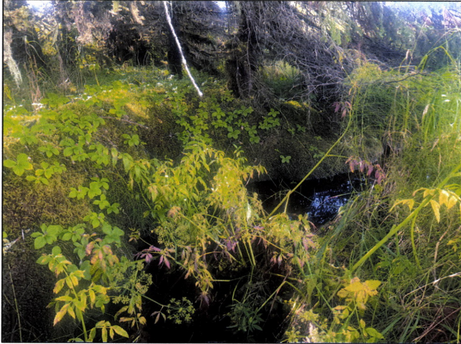
Figure 2.—Channel downstream of the culvert.
