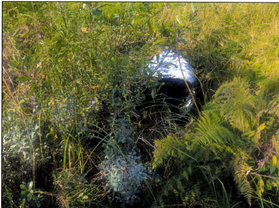
Figure 3.—Culvert upstream of the road.
