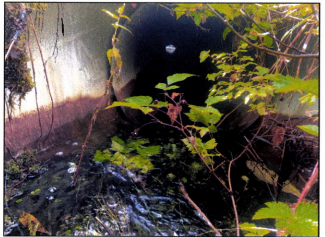
Figure 3.— Inside of culvert looking downstream.
