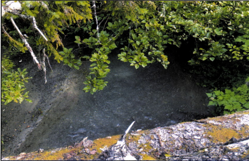
Figure 3.—Stream going under bridge at waypoint 1135, looking downstream.
