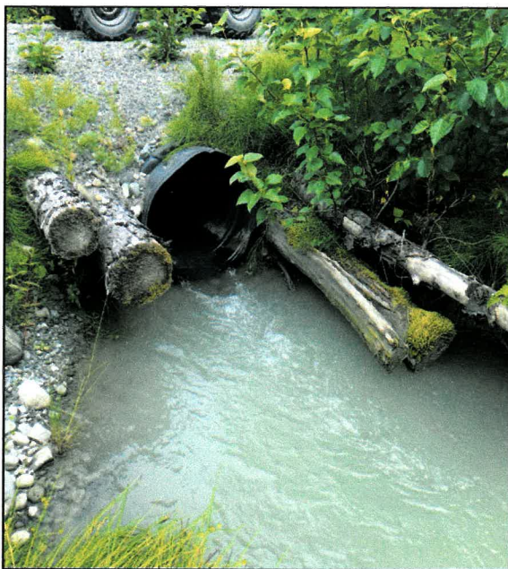
Figure 2.—Culvert outlet at waypoint 662.
