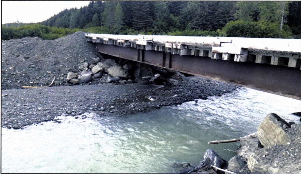
Figure 2.—West abutment of Carson Creek bridge.
