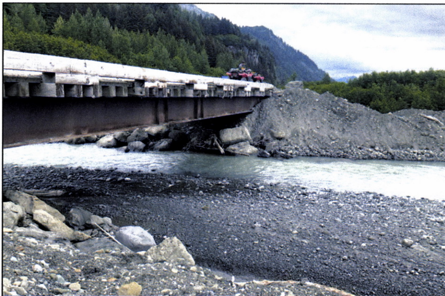
Figure 1.—East abutment of Carson Creek bridge.
