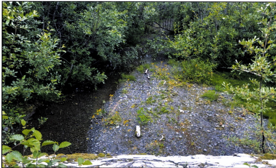
Figure 3.—Looking downstream of the bridge.
