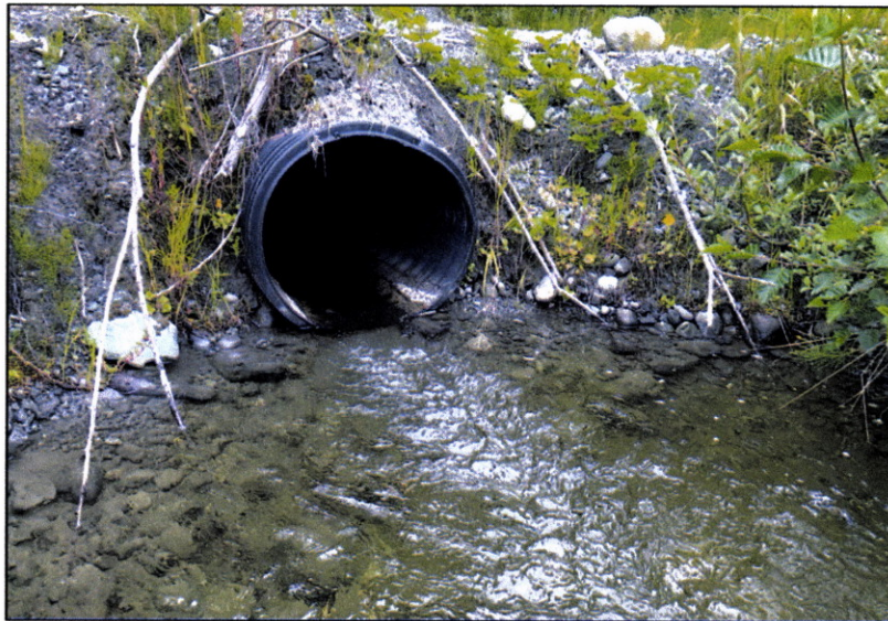
Figure 3.—Culvert outlet at waypoint 610.
