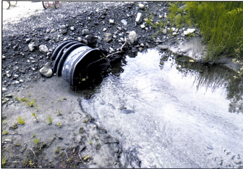
Figure 2.—Culvert inlet at waypoint 610.
