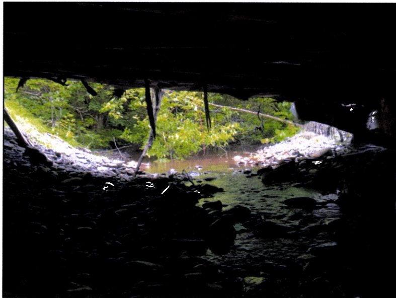
Figure 3.—Looking under bridge, downstream at waypoint 631.
