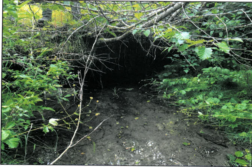
Figure 2. —Upstream of bridge, looking downstream.
