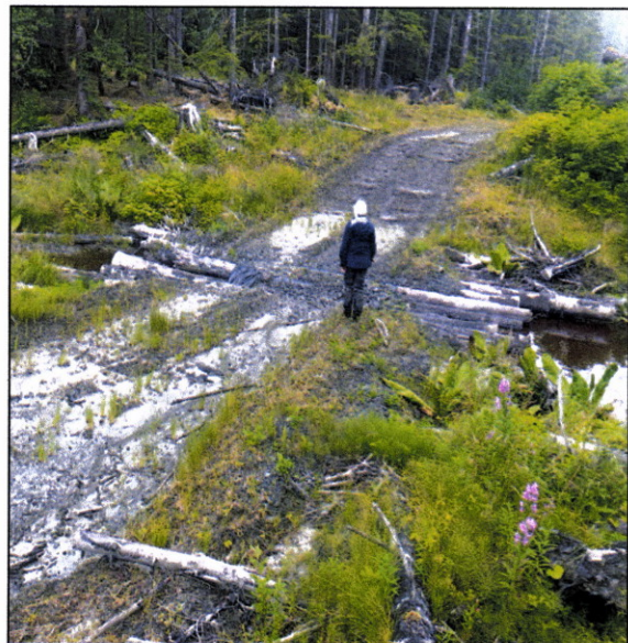
Figure 4.—Puncheon bridge at waypoint 761.
