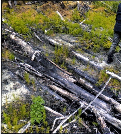
Figure 3.—Puncheon across the road at waypoint 762.
