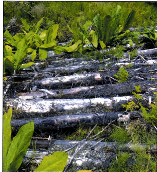
Figure 4.—Puncheon across the road at waypoint 764.
