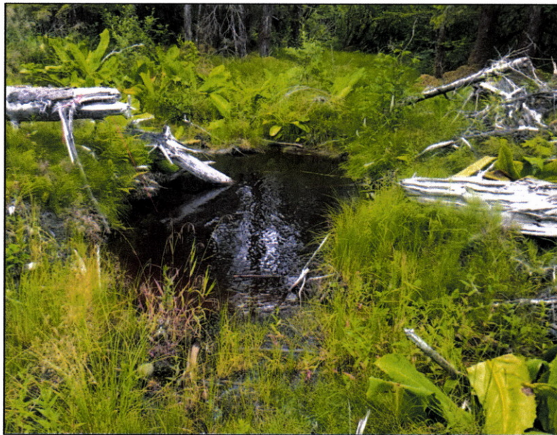
Figure 3.—Ponded water above the road at waypoint 759.
