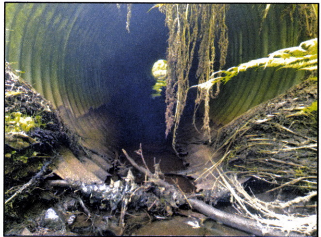
Figure 3.—Culvert just downstream of waypoint 471.
