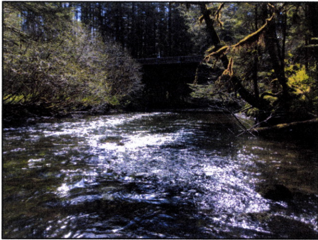
Figure 2.—Bridge at waypoint 111.
