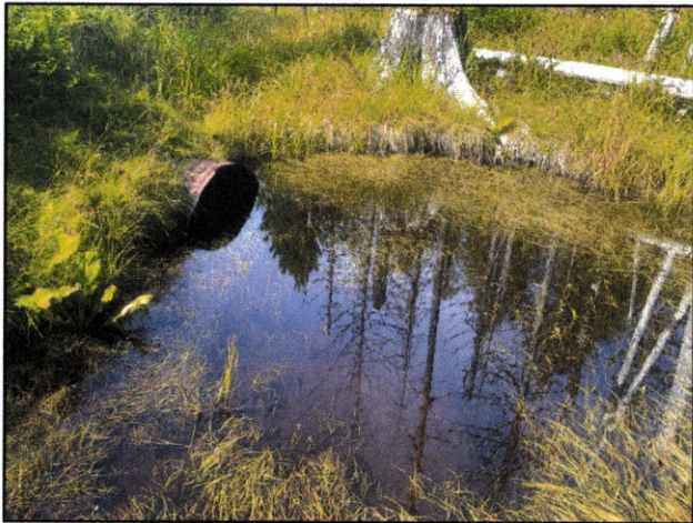
Figure 2.—Backwatered inlet of culvert at waypoint 1001.
