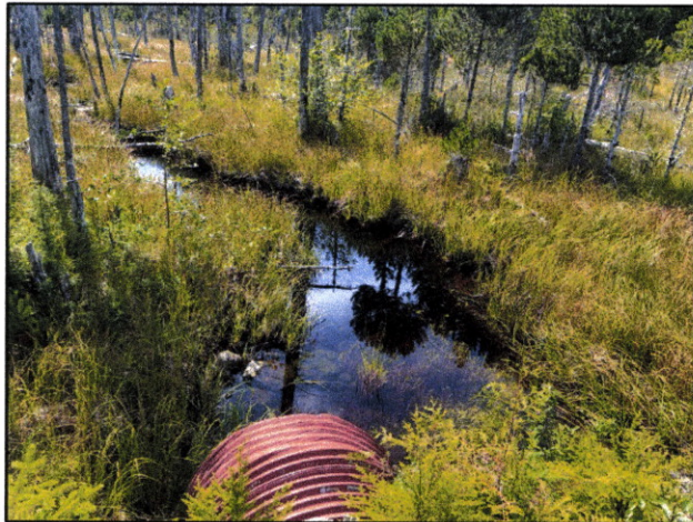
Figure 2.—Channel upstream of road crossing at waypoint 972.
