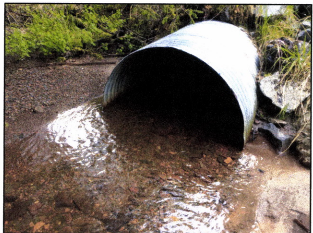
Figure 3.—Culvert at waypoint 101.
