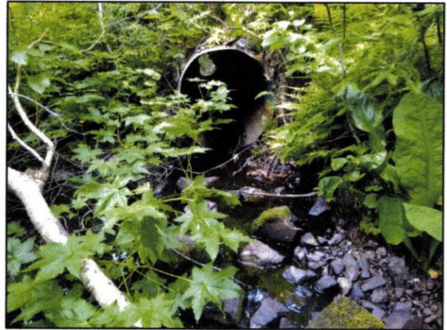
Figure 3.—Outlet of culvert at waypoint 478.
