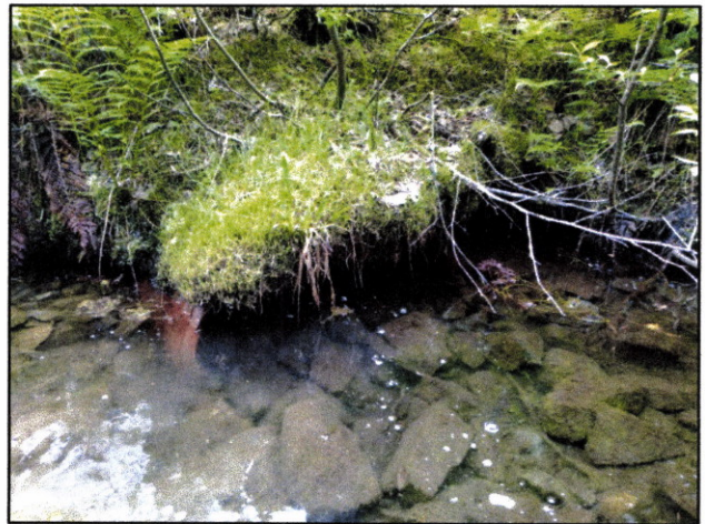
Figure 3.– Outlet of culvert at waypoint 479.
