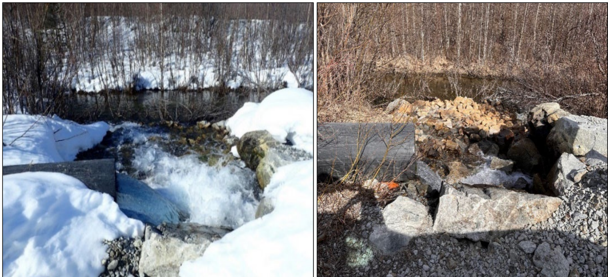
Figure 4. Outfall 002, RO water discharge of up to 3,000 gpm during 2019–2021 (2020 left) and reduced to 400 gpm during 2022–2024 (2024 right) into the RO Channel wetlands.
